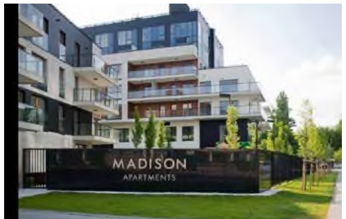
Madison Apartments - Польша - Clima Canal
